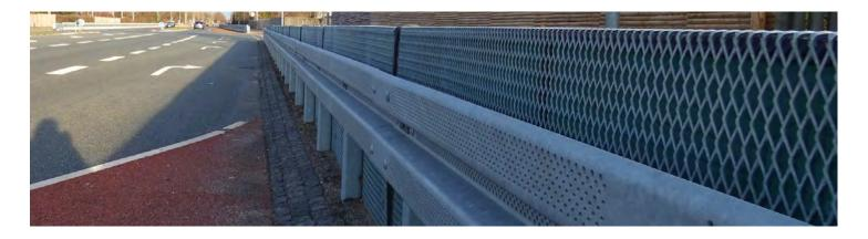
The noise absorbing guardrail system is equipped with unique perforated steel beams and special panels with stone wool filling from the market leader ROCKWOOL, that allows high noise reduction levels and impressing results in test according to the European Norm EN 14388.
