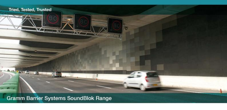
Gramm Barrier Systems TILESoundBlok® noise barrier tiles are manufactured from carefully selected specialist aggregates with angular face which are bonded together using our patented method.
