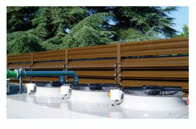
A unique design feature of the ALUSoundBlok® barrier construction is that individual panels can be removed and replaced. Panels are not bolted, welded, or otherwise permanently fastened to each other or to the support posts (Top security fixing added if required).
