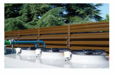
A unique design feature of the ALUSoundBlok® barrier construction is that individual panels can be removed and replaced. Panels are not bolted, welded, or otherwise permanently fastened to each other or to the support posts (Top security fixing added if required).
