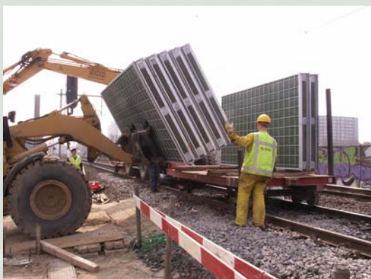
Transport of the elements to the building site
