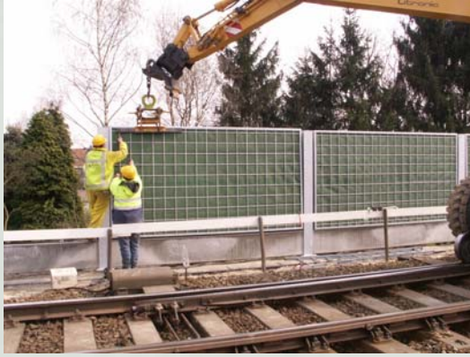
Installation of the pre assembled elements
