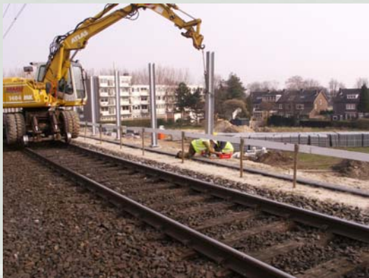
Installation of the supports from the railtrack side
