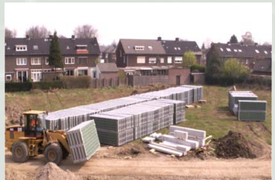
Ready elements for 2,5 km of 1,0 x 4,0 mtr
