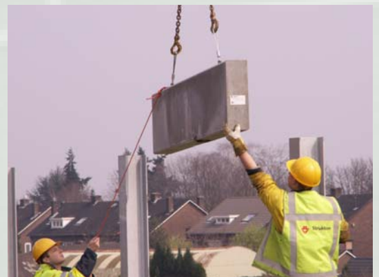
Installation of the concrete bottom part
