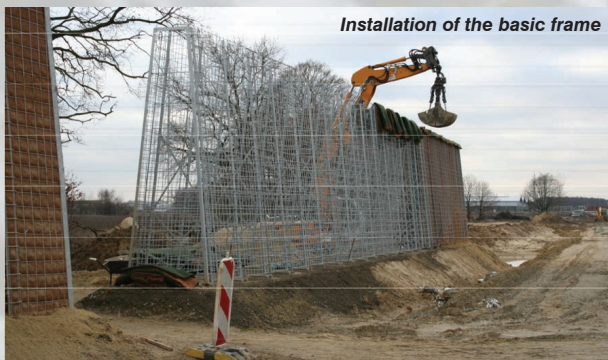
Eco barrier with coconut fibre as foundations layer
